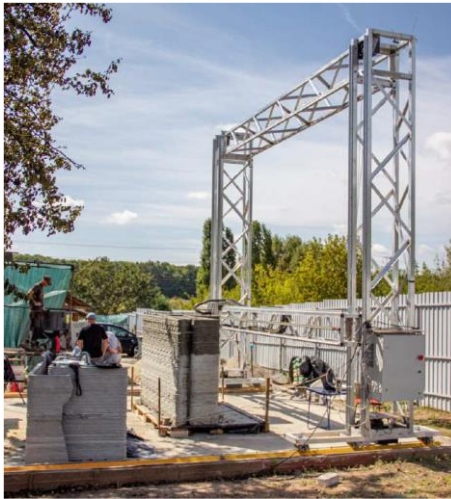
Figure 1 – Concrete 3D-printer GP-1 (manufacturer "Geopolimer" LTD, Kharkiv)
