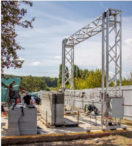
Figure 1 – Concrete 3D-printer GP-1 (manufacturer "Geopolimer" LTD, Kharkiv)
